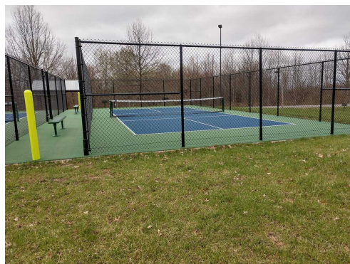
Photo: Matéflex helped Marcy convert tennis courts into pickle ball courts.
